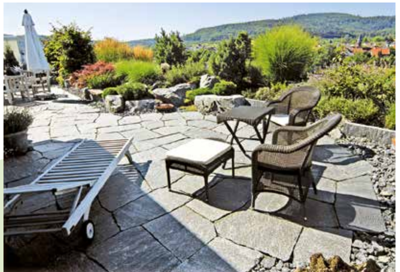
Intensive Green Roof
